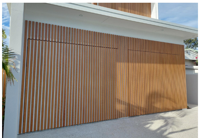
Flush Mount Tilt door with Knotwood battens
