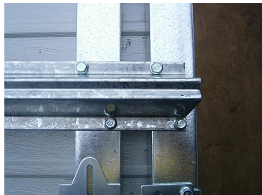
Figure 4 – Typical strut fixing pattern for all stiles.
