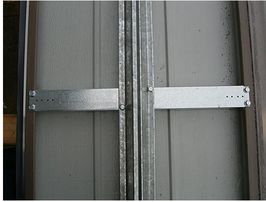
Figure 7 – Typical Strut & Stile Fixing
