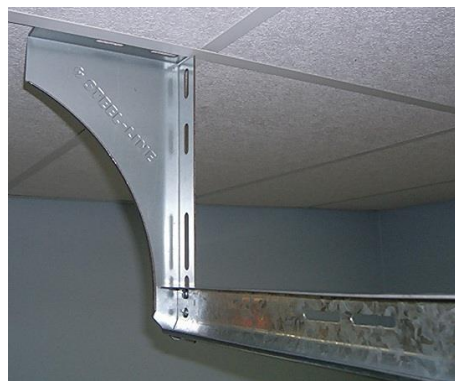
Figure 10 – Typical Rear Track Hangers for End of 2400 Horizontal Track (Optional Horizontal Track Bracket shown)
