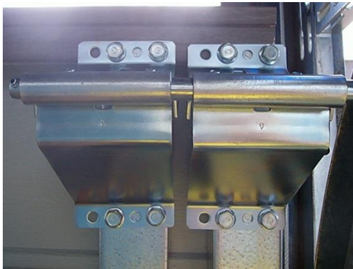
Figure 14 – Top Bracket Mounting
