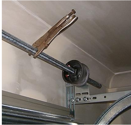
Figure 16 – Clamping Shaft Prior to Spring Tensioning (vice-grips resting against ceiling in this case)
