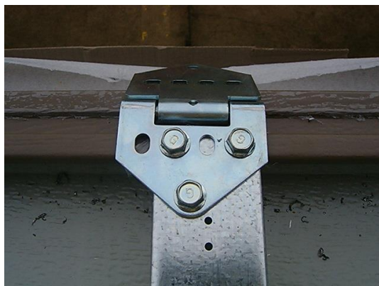
Figure 6 – Typical Centre/Intermediate Hinge Fixing
