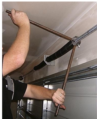
Figure 17 – Tensioning Springs
