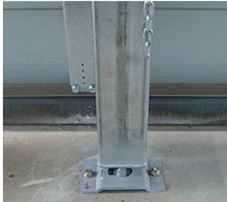
**STEP 3:** Lift top inner post and fix to wall bracket, by removing the pin, inserting top arm into bracket clevis and re-installing the pin.
