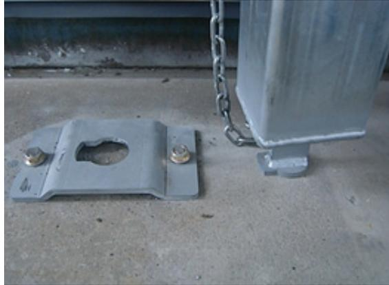
**STEP 2:** Rotate post in base plate ¼ turn so that top arm faces wall bracket. Secure post temporarily to a stile using the chain from one of chain brackets (this prevents post falling over while doing Step3).
