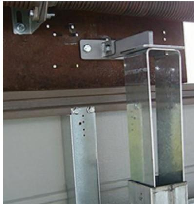
**STEP 4:** Feed chain under & over strut & hook back onto chain bracket. Repeat for all post to strut connections.
