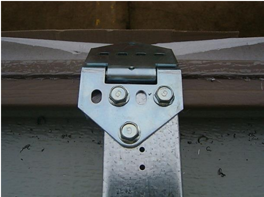
Figure 2 – Typical Centre/Intermediate Hinge Fixing
