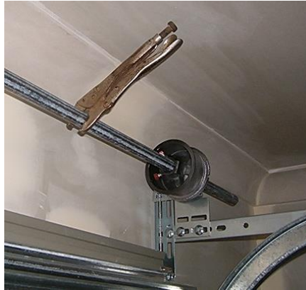
Figure 8 – Clamping Shaft Prior to Spring Tensioning (vice-grips resting against ceiling in this case)
