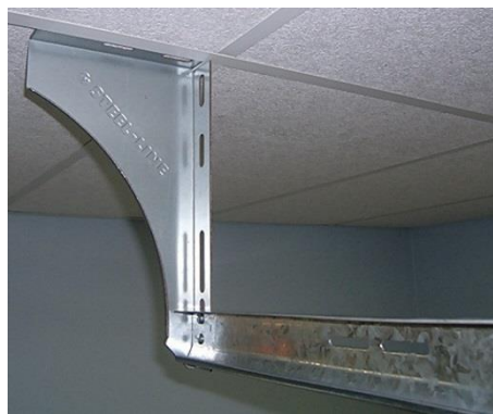
Figure 5 – Typical Rear Track Hangers for End of Horizontal Track
