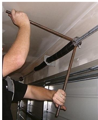
Figure 9 – Tensioning Springs
